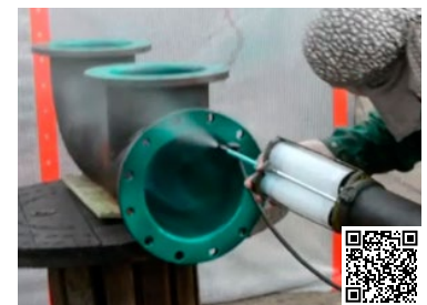
Video 21.4 Spraying technique for overhead applications
