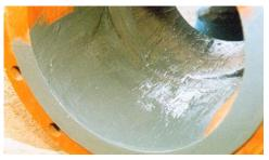
The daily repair routine when epoxy ceramic compounds are used for linings. No hydraulic engineer wants to see irregular surfaces like this ...
