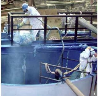
MetaLine® meets heavy duty off-shore corrosion protection standards. Electro-chemical anodic properties combined with a rubberlike atmospherical encapsulation surpasses over 6,000 hours saltspray-chambertest as per ASTM. Withstands up to 70 bar (1,000 psi) of water pressure.
