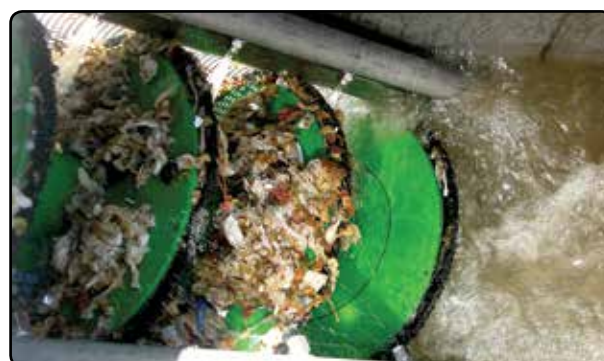
Solids captured and removed by auger
