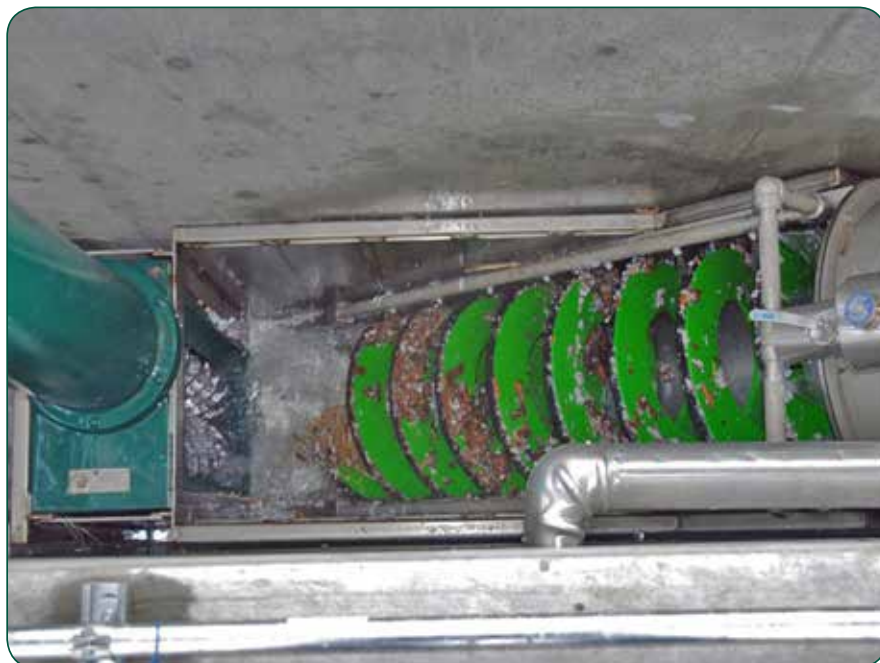
Debris is Washed and Lifted to the Discharge Point via Spiral Lift
