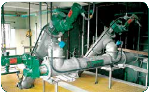
Auger Monsters and cross conveyor
