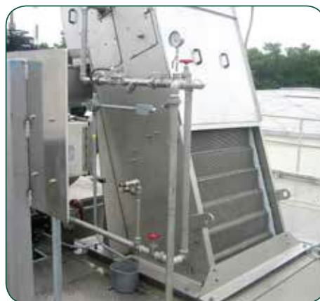
Solids are captured on the perforated panels and conveyed to the discharge level.
