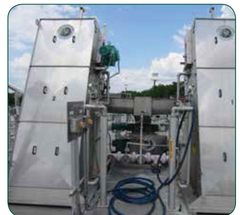
Dual Finescreen Monster removing solids and feeding a sluice
