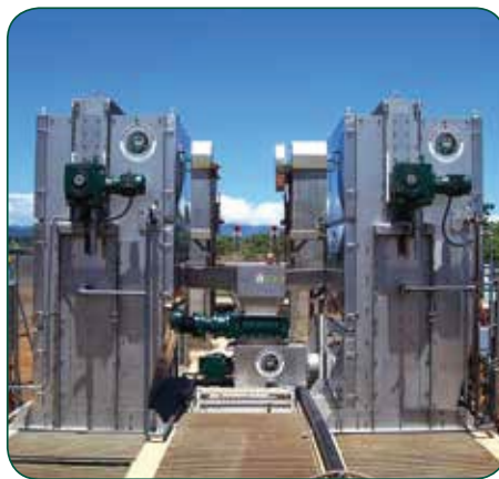
A pair of Bandscreen Monsters operating at a wastewater treatment plant in Hawaii.
