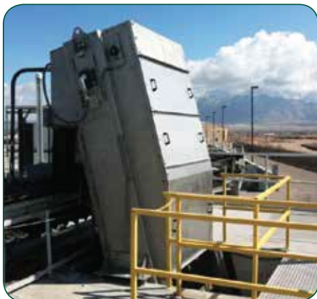
Completely enclosed above operating floor level with easy to remove stainless steel guards
